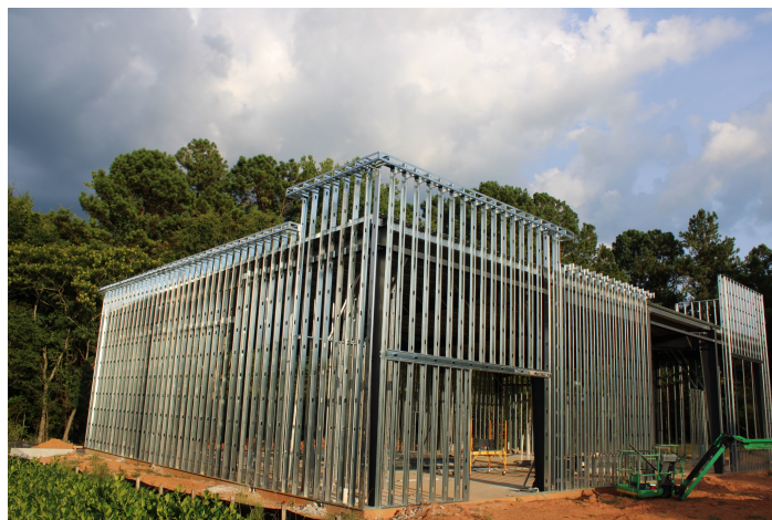
Figure 2: Cold Formed Steel Framing
