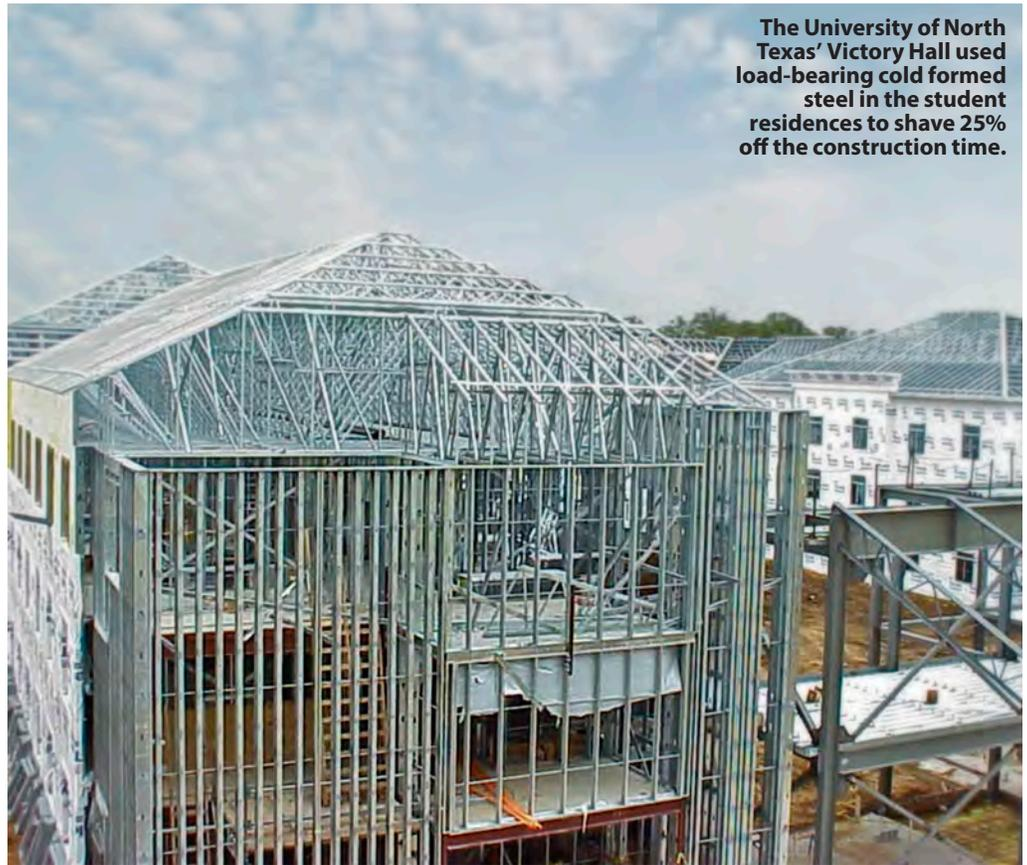
The University of North Texas' Victory Hall used load-bearing cold formed steel in the student residences to shave 25% off the construction time.
