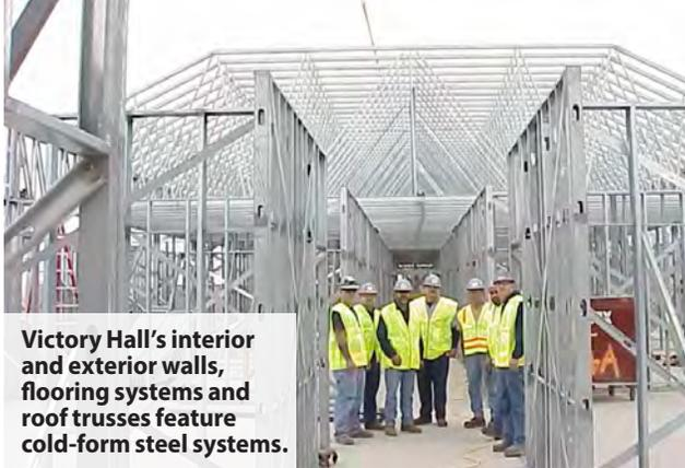
Victory Hall's interior and exterior walls, flooring systems and roof trusses feature cold-form steel systems.
