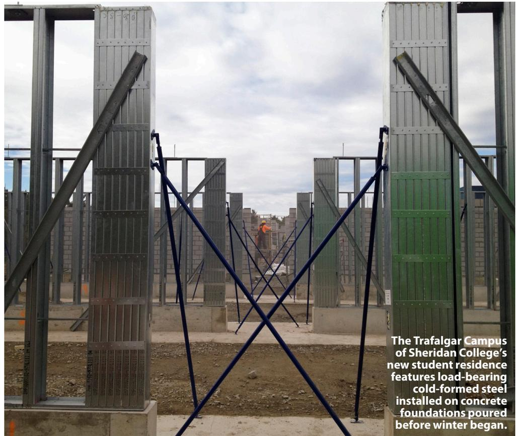
The Trafalgar Campus of Sheridan College's new student residence features load-bearing cold-formed steel installed on concrete foundations poured before winter began.
