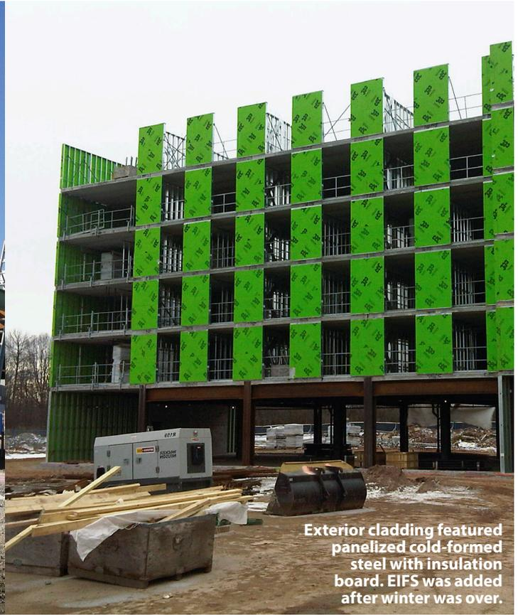
Exterior cladding featured panelized cold-formed steel with insulation board. EIFS was added after winter was over.
