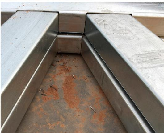
Each truss was assembled with 350 self-tapping screws. All parts were ink-jet labeled to make on-site assembly easy.
