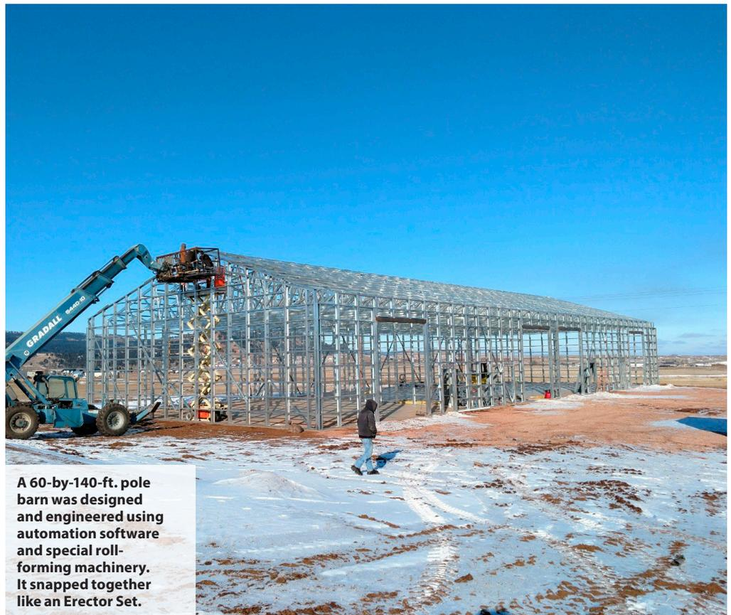
A 60-by-140-ft. pole barn was designed and engineered using automation software and special roll-forming machinery. It snapped together like an Erector Set.
