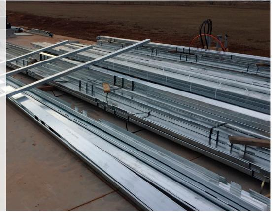
Notching enabled truss webs to slide into position. No welding or re-galvanizing was needed.
