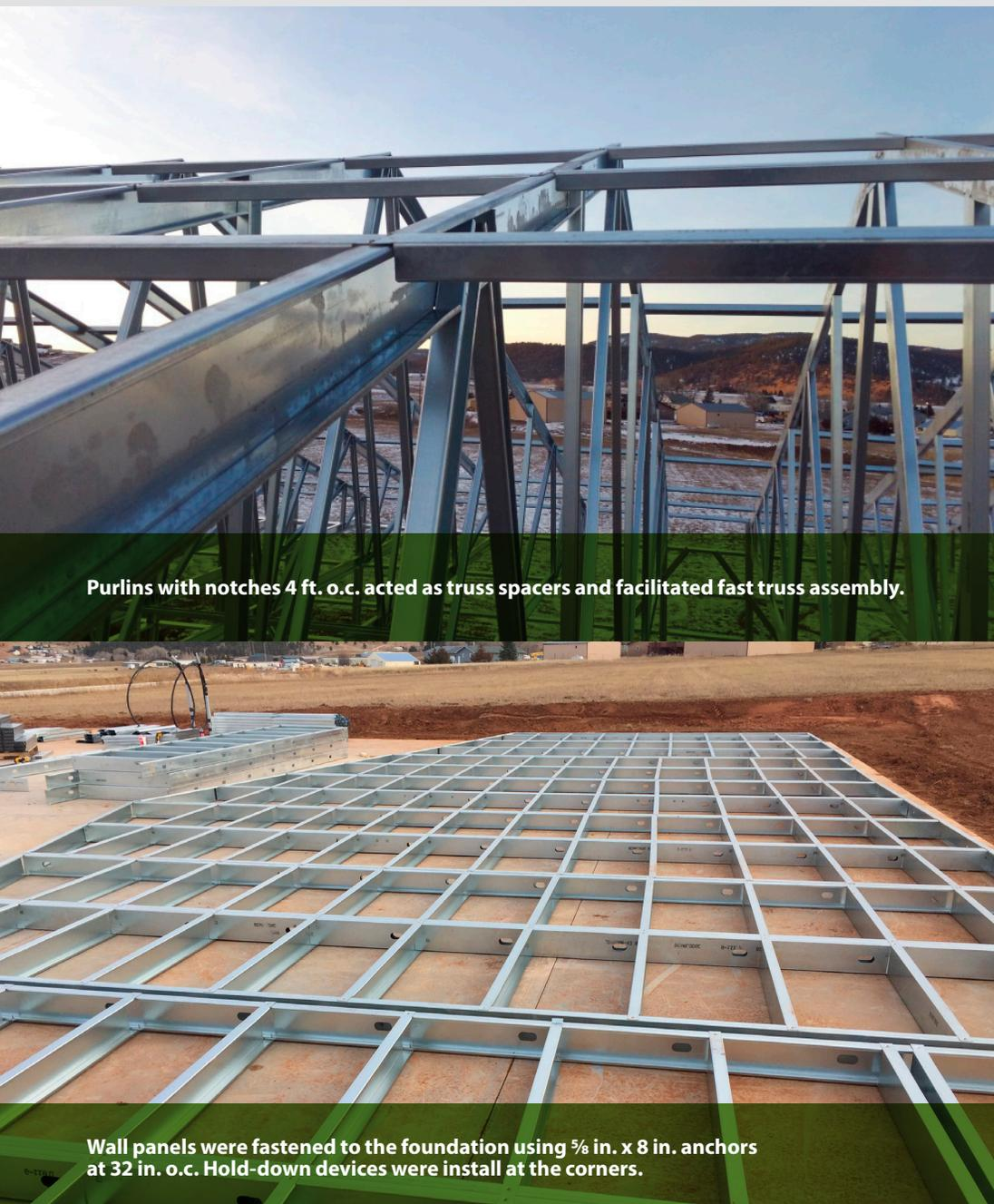
Purlins with notches 4 ft. o.c. acted as truss spacers and facilitated fast truss assembly.
