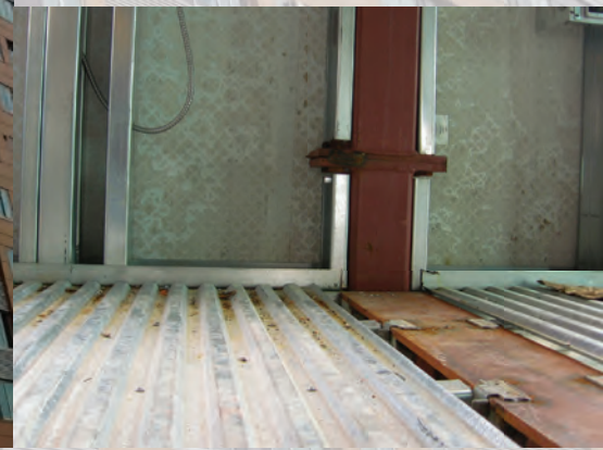
Hot-rolled steel was used strategically only for the first two floors.
