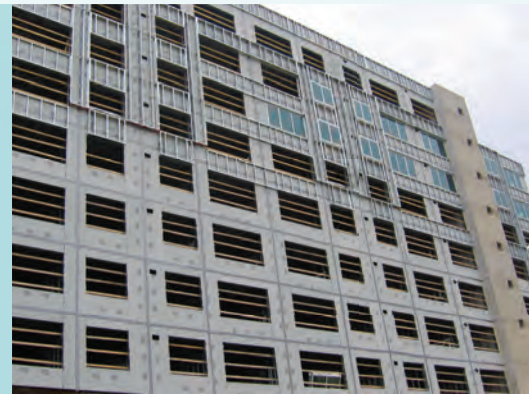
Exterior cold-formed steel framing is the primary load-bearing system for the top eight floors.
