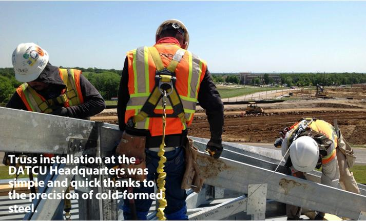
Truss installation at the DATCU Headquarters was simple and quick thanks to the precision of cold-formed steel.
