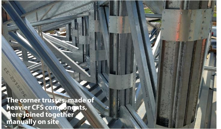
The corner trusses, made of heavier CFS components, were joined together manually on site
