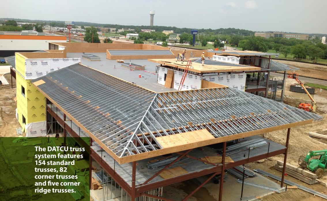
The DATCU truss system features 154 standard trusses, 82 corner trusses and five corner ridge trusses.
