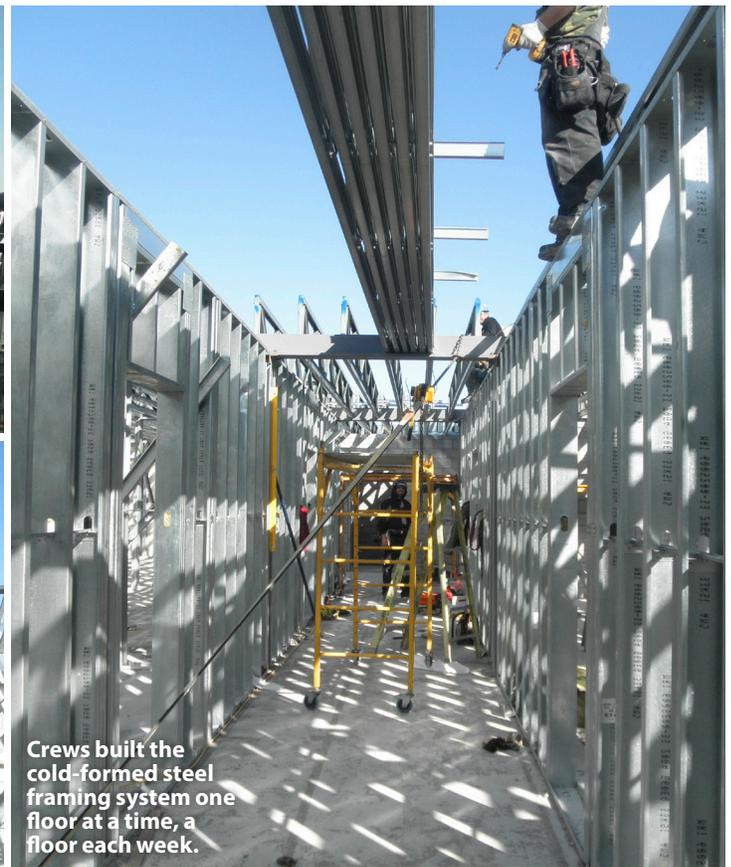
Crews built the cold-formed steel framing system one floor at a time, a floor each week.
