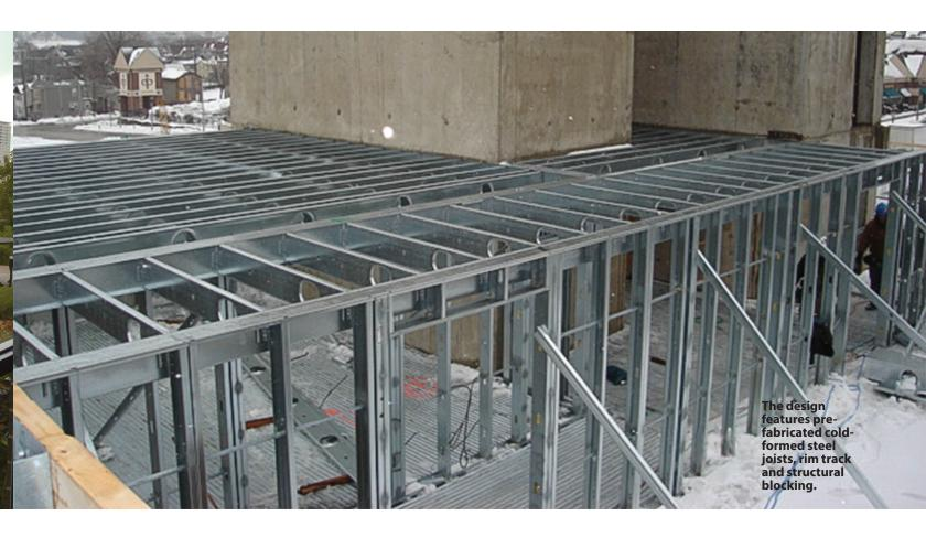
Matsen Ford Design Associates, Waukesha, Wis., engineered the project's cold-formed steel system, which comprises the majority of the structure's support system.
