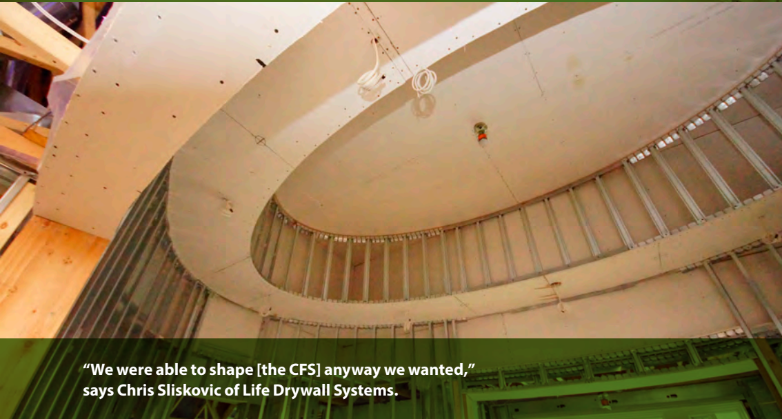
Bay windows feature CFS posts, lintels, sills and connections.
